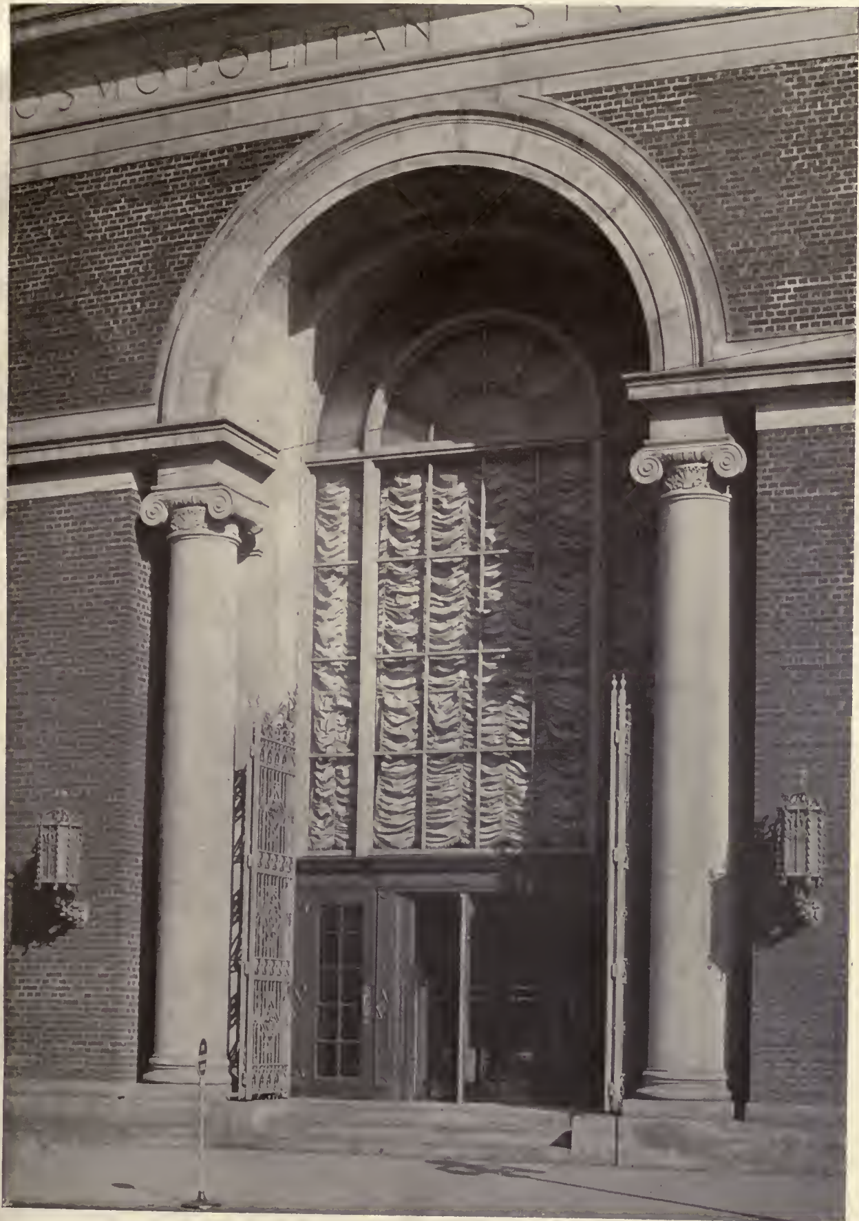
DETAIL OF MAIN ENTRANCE COSMOPOLITAN STATE BANK, CHICAGO, ILL. RICHARD E. SCHMIDT, GARDEN & MARTIN, ARCHITECTS
